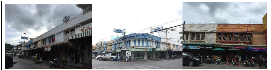
Figure 111: Commercial buildings around Chatchai Market on 26 Sep 2016
