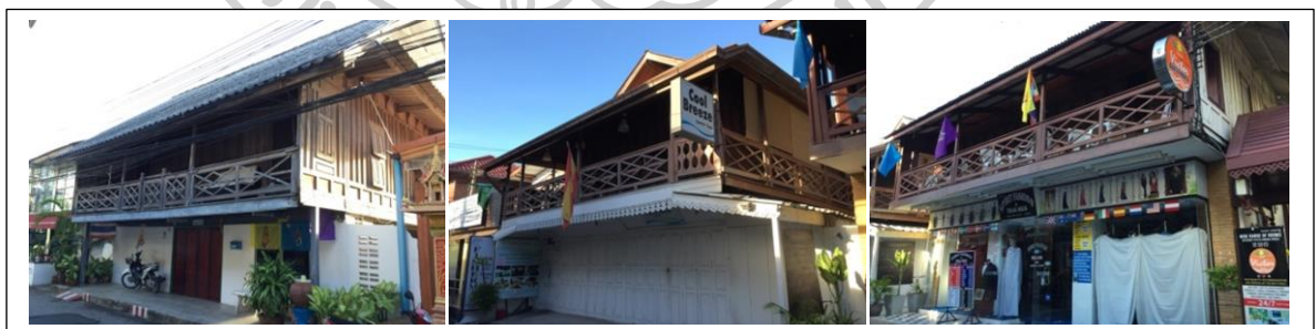
Figure 60: Houses & tailor shop on Naresdamri Road
