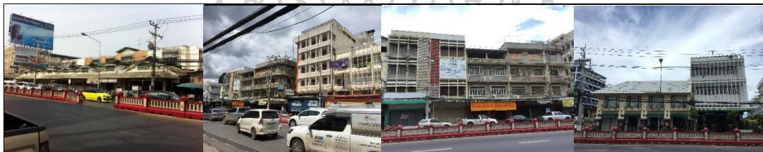
Figure 112: Commercial buildings around Chatchai Market on 26 Sep 2016
