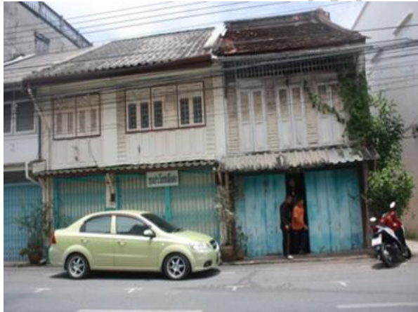
Figure 35: Old building design in the old town area Source: Ms. Yingrak Chakcharoen (July 2016)
