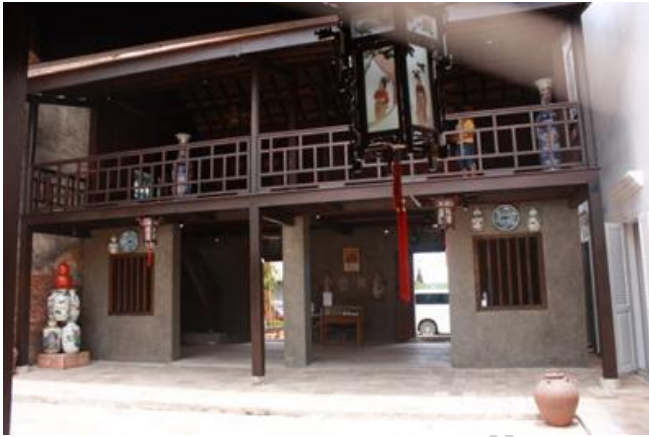
Figure 34: Old building design in an old town area Source: Ms. Yingrak Chakcharoen (July 2016)
