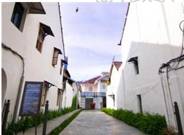
Figure 79: The entrance of Chulia Heritage Hotel
