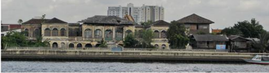
Figure 32 Praya Palazzo before renovation
