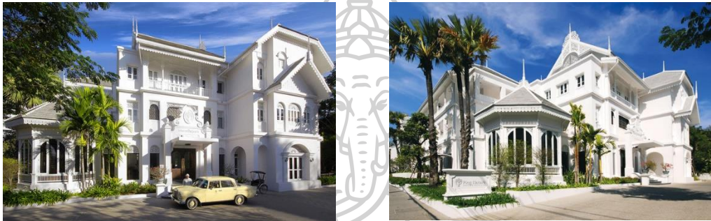
Figure 37 Exterior of Ping Nakara
