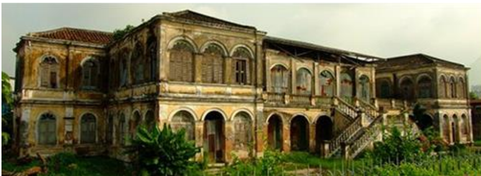
Figure 31 Praya Palazzo before renovation
