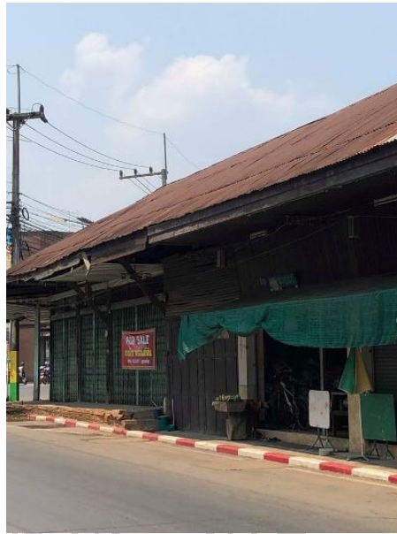
Figure 38: Old houses in Si Phanom Mat without description of heritage values Source: Photo taken by the author, 17 March 2018
