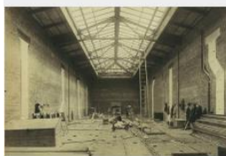
Construction of the West Gallery, 1913
