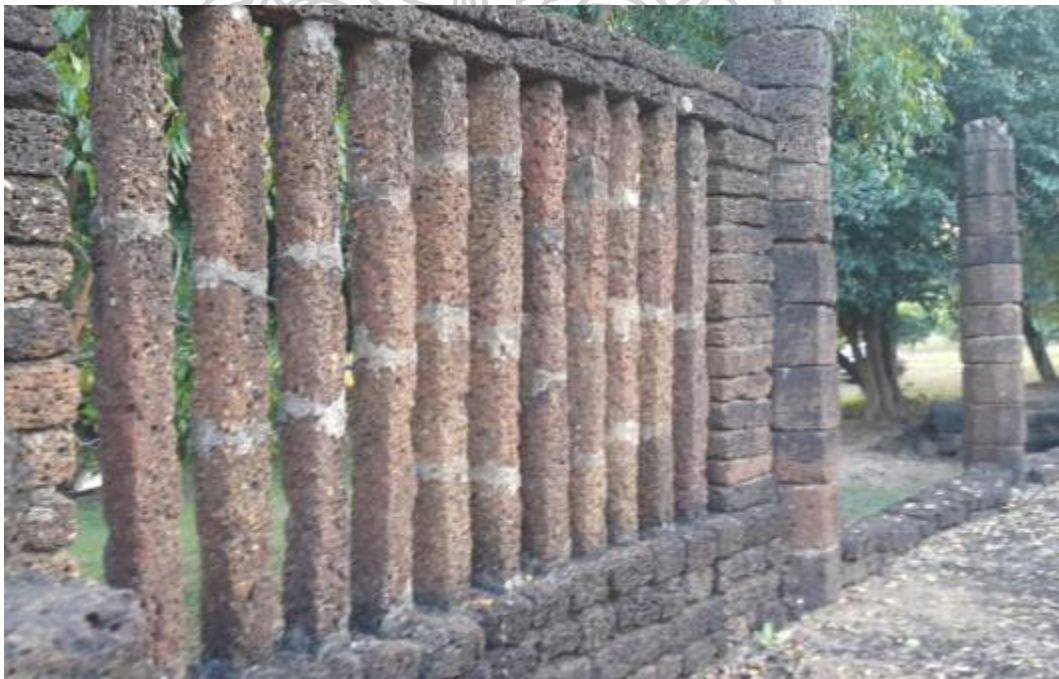
Figure 163: The wall detail of Wat Yai Ta
