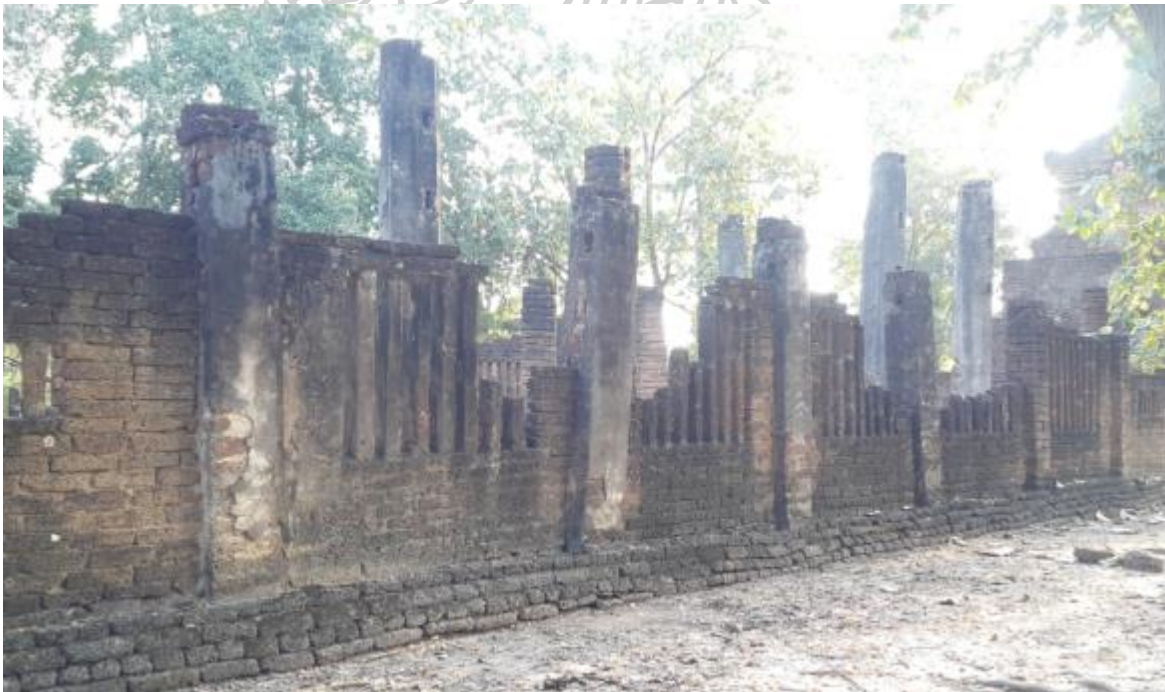
Figure 157: The wall detail of Wat Rahu
