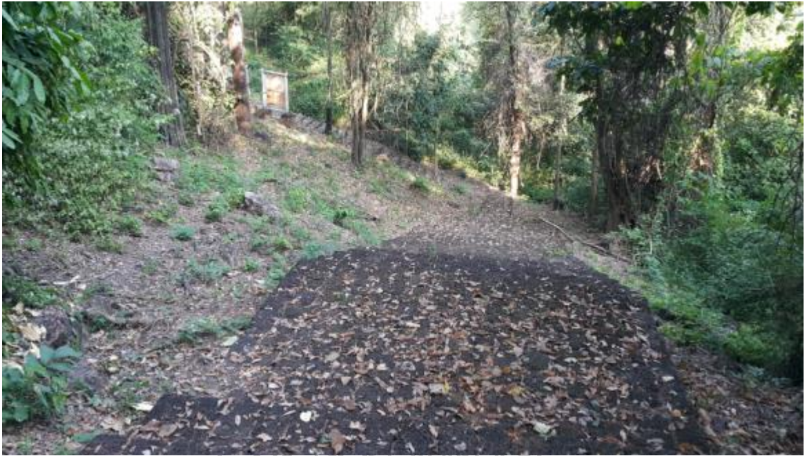
Figure 137: The slope of the historical site that has no rails
