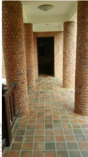
Figure 30: Pathway that links the buildings is surround with beautiful garden
