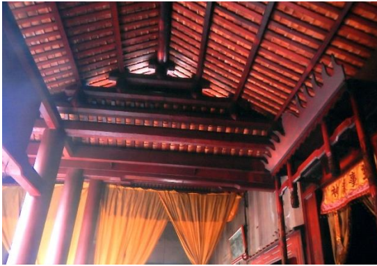
Figure 186: Cha Liang, insert crossbeam, in Kew Ong Ear Shrine.
