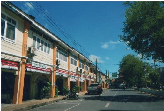
Figure 309 : Peranakan Chinese Shophouses on Buriwanit Road.
