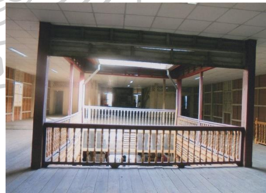
Figure 302 : The second storey of the building.
