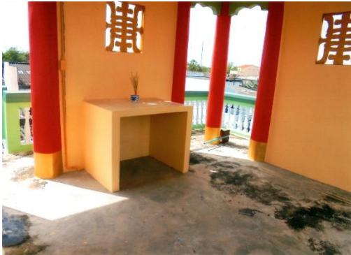
Figure 205 :The third storey of the building.
