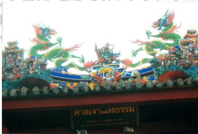
Figure 174: The roof of Sang Tham Shrine after renovation in 2004.
