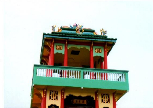
Figure 206 :The roof of three-storey building of the shrine.
