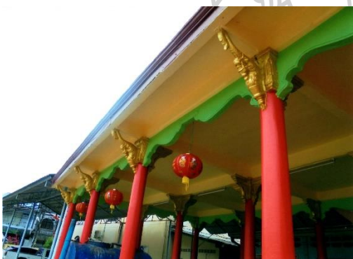
Figure 203 :The Thai style corbels of Chinese dragons on the row of the first storey of the building.
