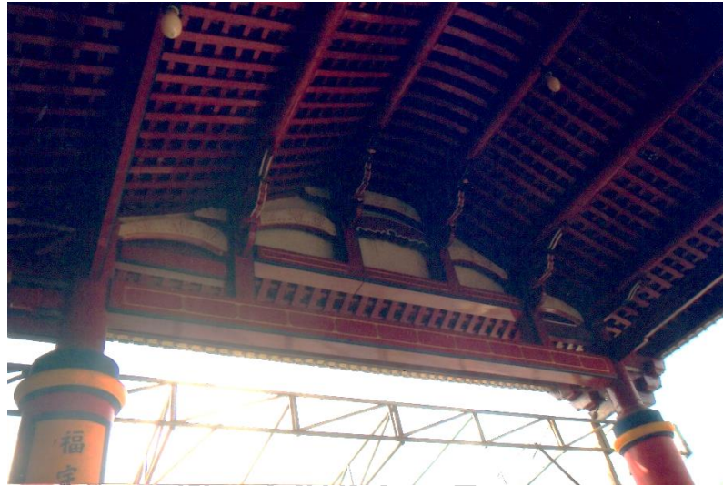
Figure 147: "Chaliang", insert crossbeam, at Mazhu Shrine, Phang-nga City.
