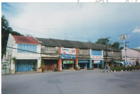
Figure 303 :Ong Tong Guan's Peranakan Chinese Shophouse at the end of the row of Peranakan Chinese Shophouses in Kantang Town.
