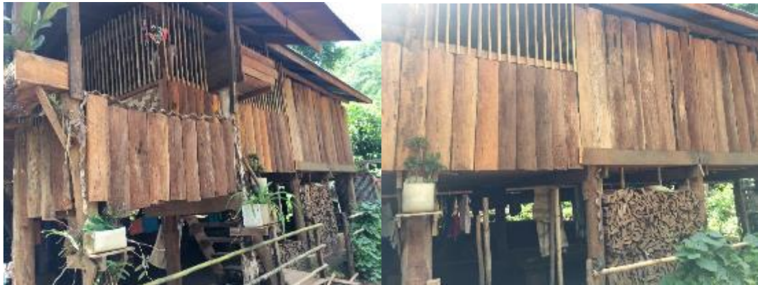
Figure 49 The Kayan house within Ban Huay Pu Keng which is built in the Thai rural style
