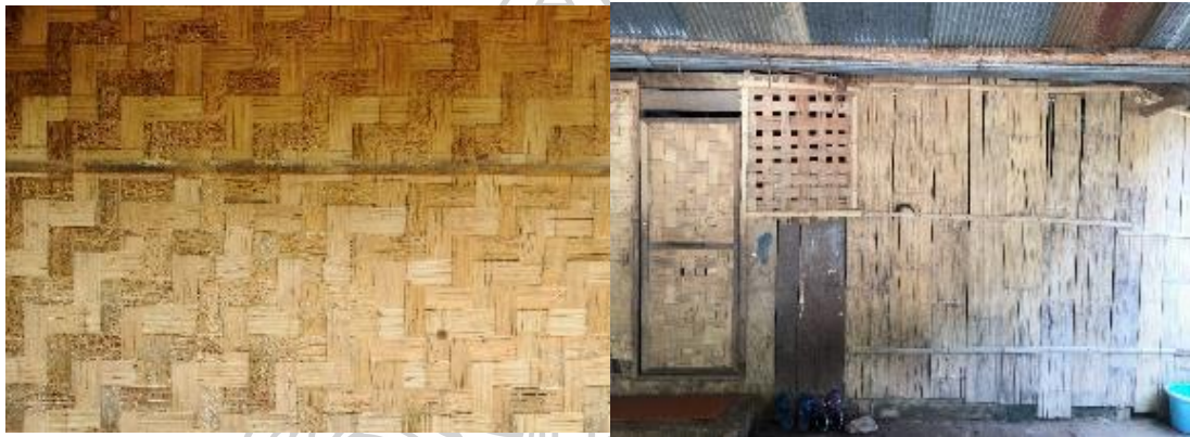
Figure 45 The pattern of walls which are woven split bamboo
