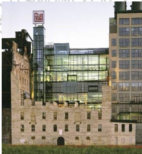
Figure 20 Architectural Integration of New Section with Old into a Museum Source: https://plus.google.com , 2013.
