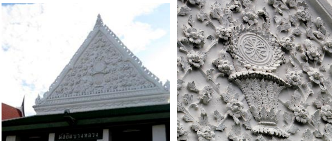
Figure 123 Stucco Pattern Decoration at the Pediment
