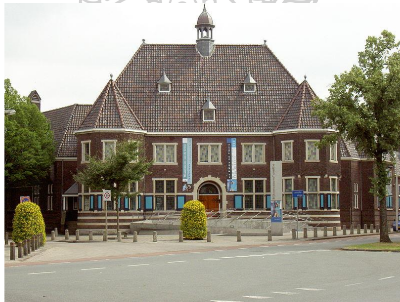
Figure 14 Old Building of Rijksmuseum Twenthe Museum Source: www.asla.org , (American Society of Landscape Architects., 2013).
