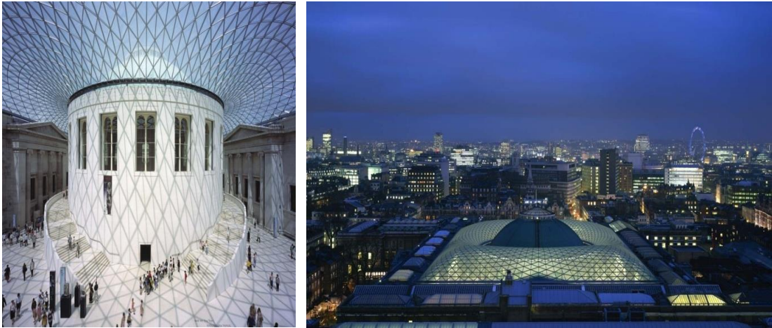
Figure 4 The Vast Glazed Canopy Expressing Ancient Atmosphere in a Court Type in the Roman Era by Modernized Construction Technology Source: Norman Foster and partners, (Foster et al., 2001)
