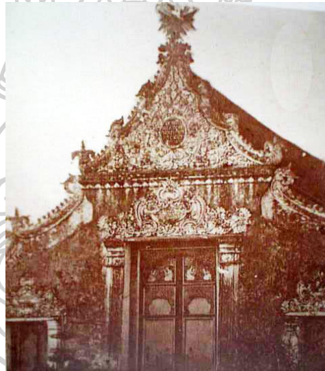
Figure 86 Picture of the Second Building of the Church
