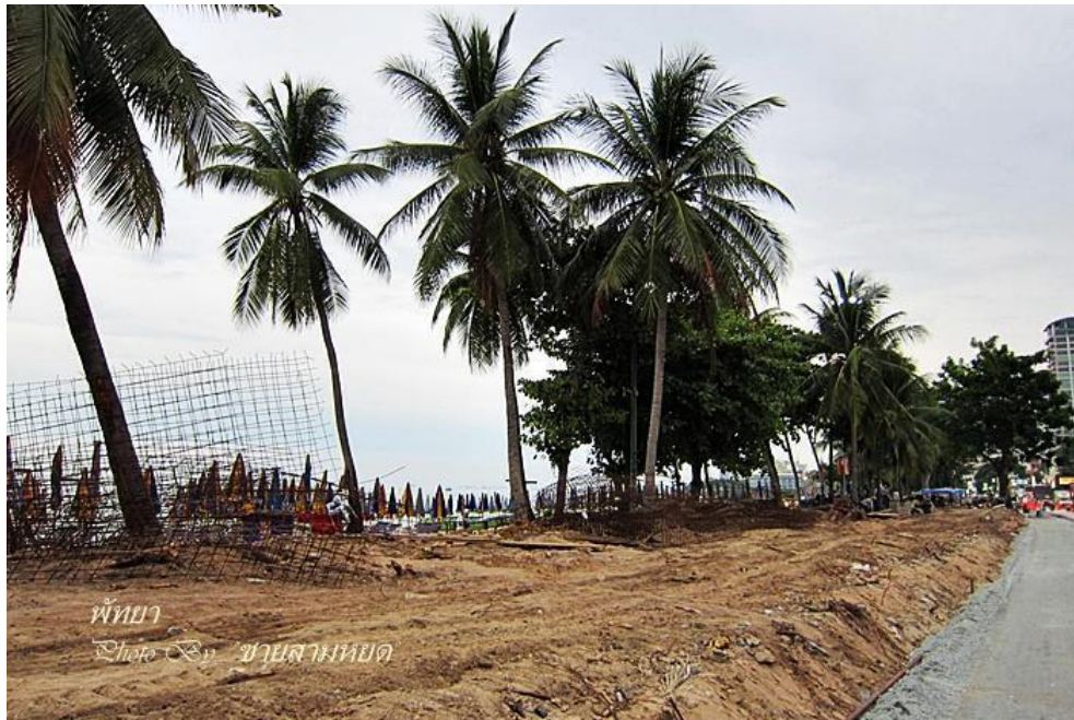
Figure 12: Pattaya beach road during the reconstruction
