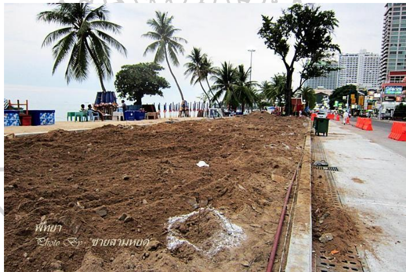
Figure 3: Pattaya beach road during an improvement
