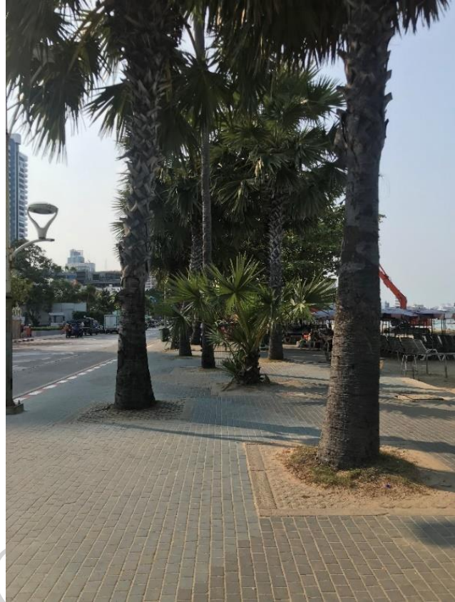
Figure 14: Pattaya beach road after the reconstruction
