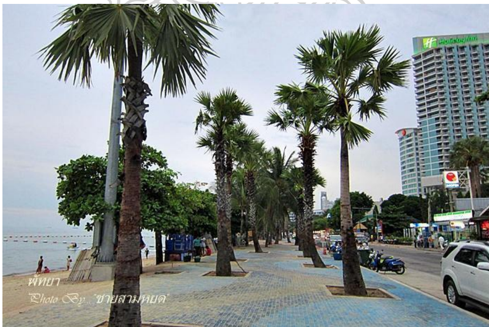
Figure 13: Pattaya beach road after the reconstruction
