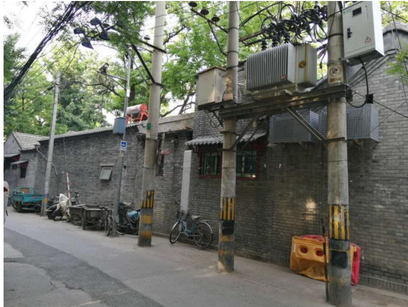
Figure 36 The grey walls extend along the street, and the telegraph poles crisscross the walls, creating an aesthetic of chaos.
