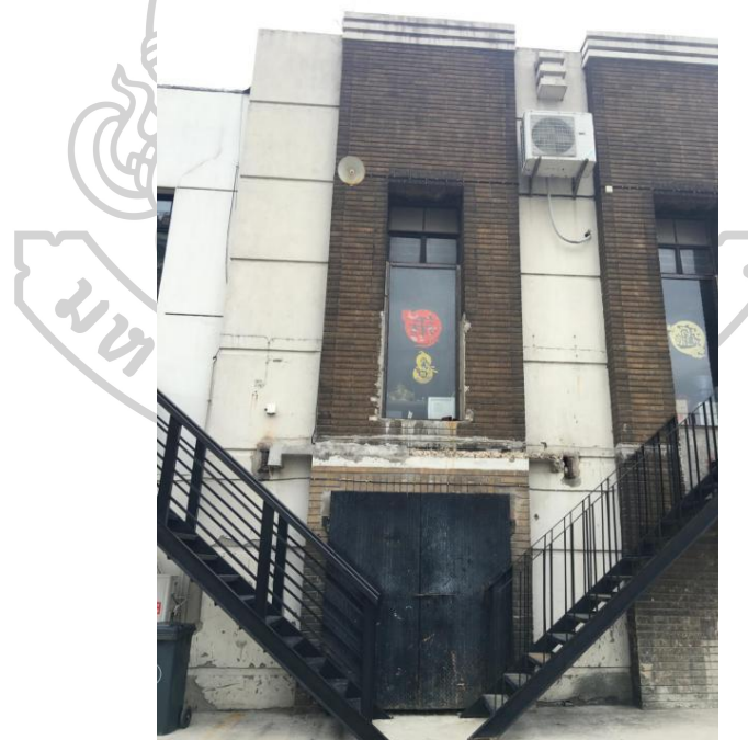
Figure 44 Windows in modern architecture are more diversified and practical. Source: Shot by the author in Shanghai, China, March 2018.
