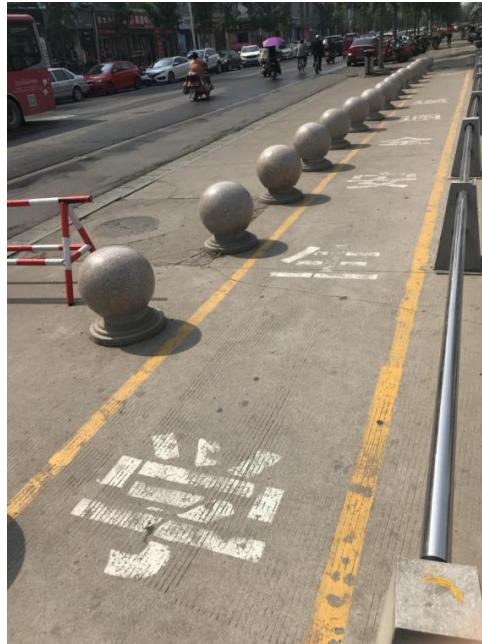
Figure 78 In order to ensure road safety, the Chinese government has set up road logos on the ground for students' safe passage.
