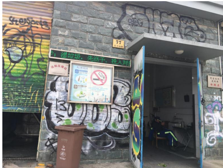
Figure 26 Functional doors of modern architecture can also be combined with other art forms to present a hard aesthetic.
