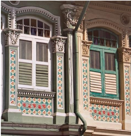
Figure 59 Tiles at façade (Knapp, 2012, p.24).
