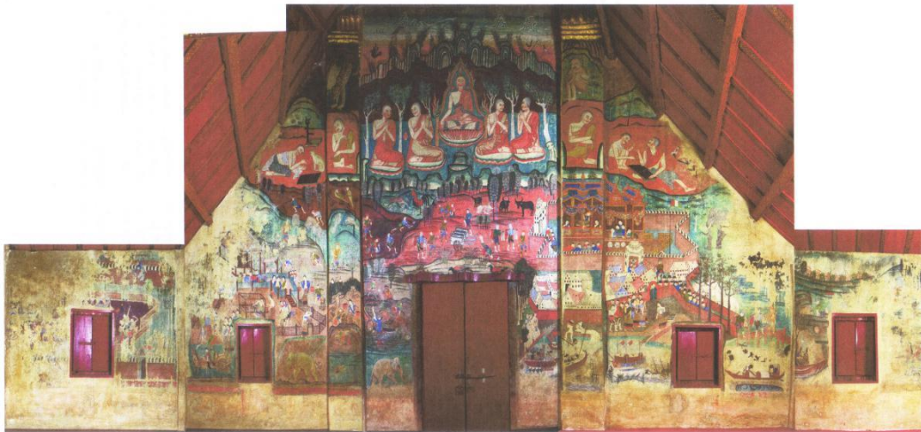
Figure 52 Photograph of North side of the wall at Wat Phumin, Nan province Source : Pattana Decha
