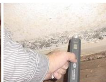
Taking specific damp meter readings
