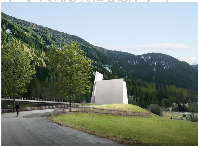
Figure 100 New Motorway Chapel for Switzerland A13 road (Baldwin, 2020)
