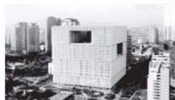
Amorepacific Headquarters / David Chipperfield
