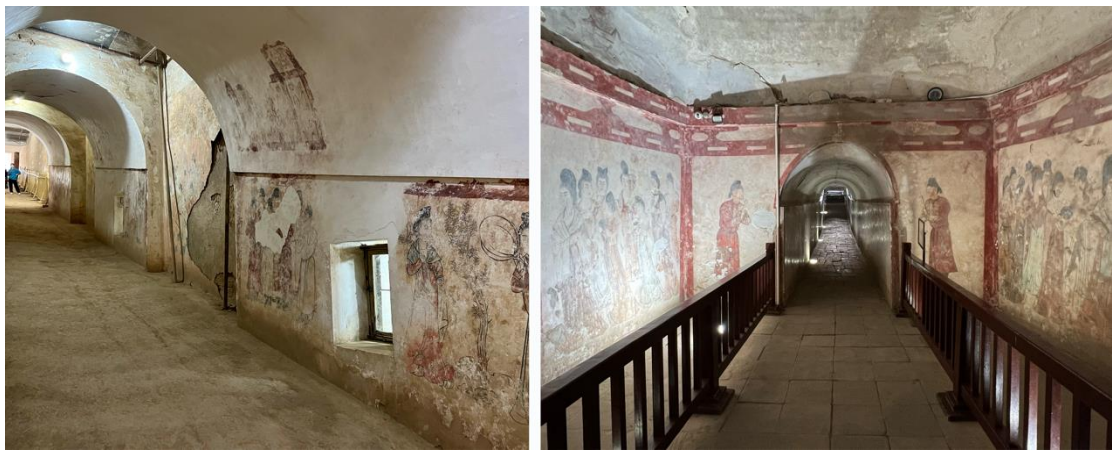
Figure 78 The structure of the mural tomb in the Tang Dynasty Source: Photographed by the Author, 2021.
