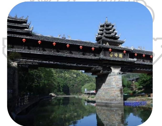
Figure 45 Hunan Huangdu General Repair Fengyu Bridge
