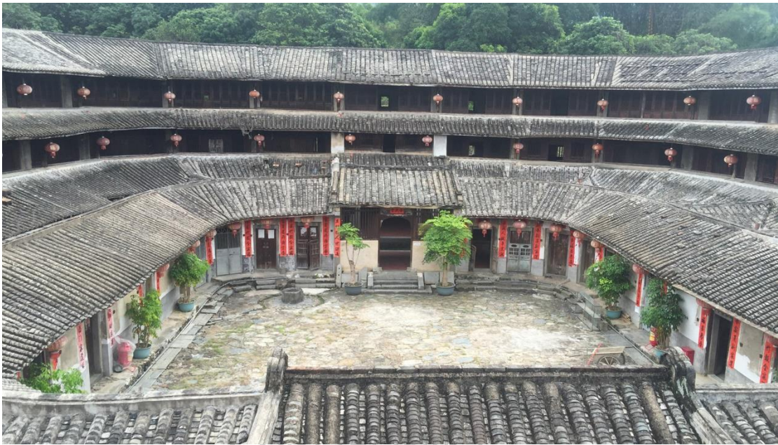
Figure 53. Slightly Damaged, Lanwucun Source: Author (2022)
