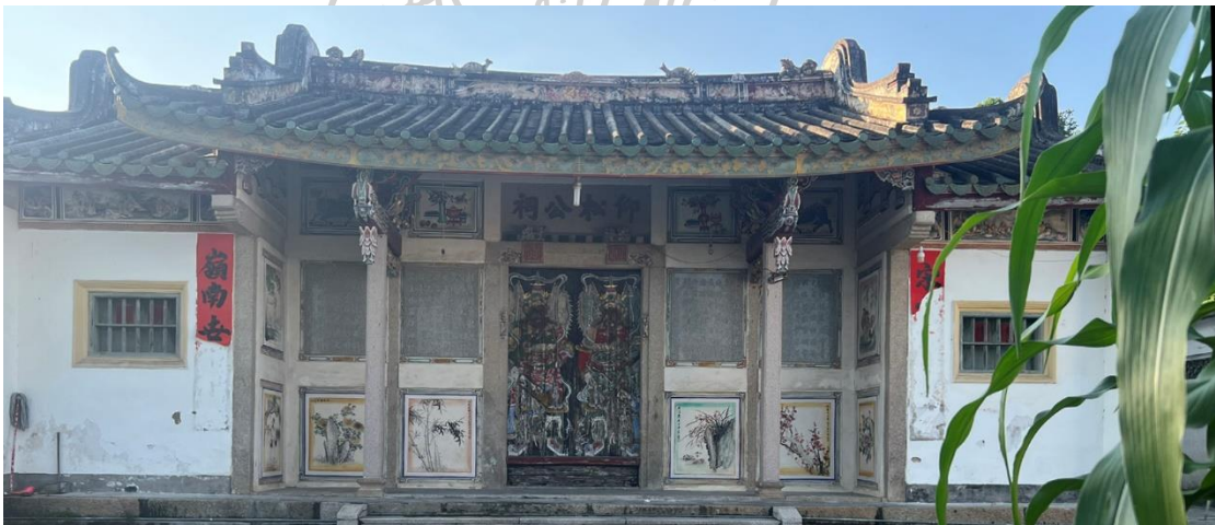
Figure 54. Good Condition, Woshicun Source: Author (2022)
