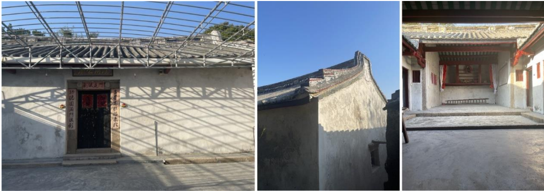
Figure 122. Good Condition Buildings, Woshicun
