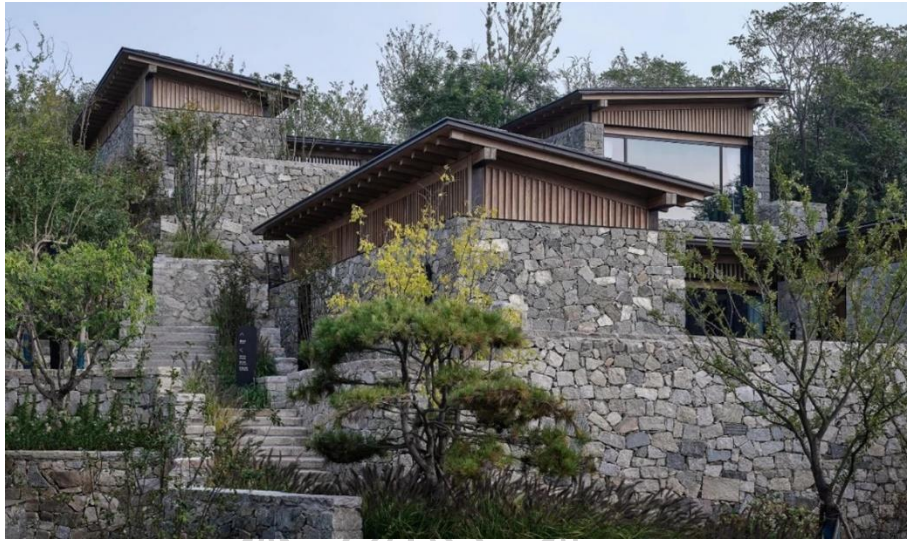
Figure 31. Courtyard No. 7, Tai'an Dongximen Village
