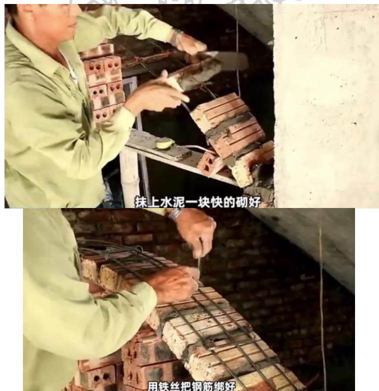
Figure 13: the making of an arch door frames
