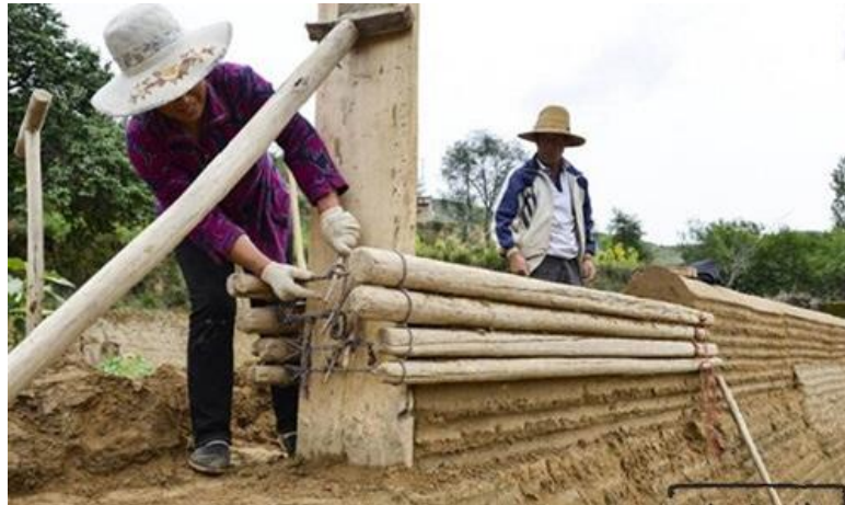
Figure 31: Build rammed earth walls
