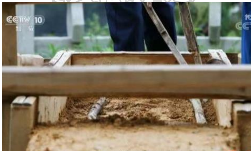
Figure 11: Putting in bamboo sheets to press the earthen wall
