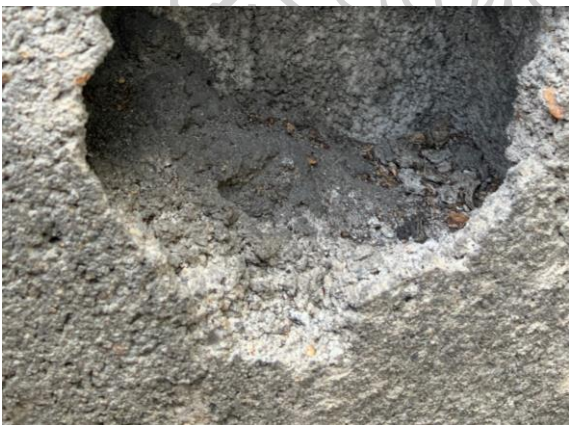
Figure 66 Dust and dirt accumulate in the hollow space of the concrete block Source: Khakhanang Jonganurak (June 12, 2023)
