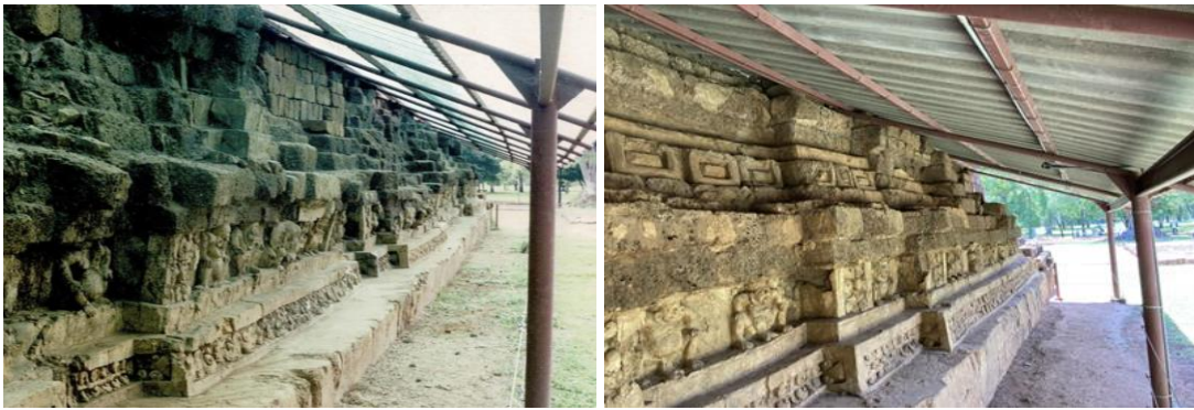
Figure 82 The transparent shelter for the stucco of the Khao Klang Nai
