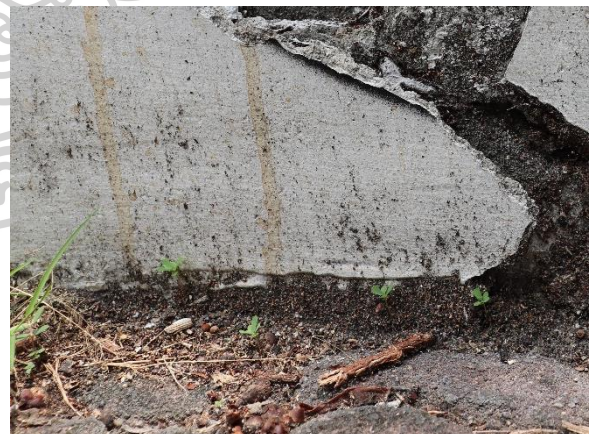
Figure 76 Peeling of paint layer on the drilling mark Source: Khakhanang Jonganurak (January 16, 2023)
