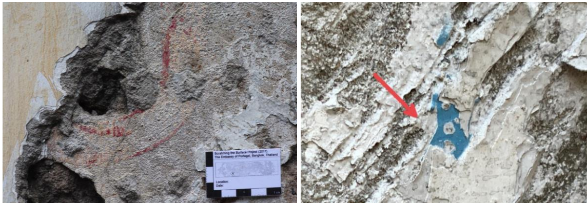
Figure 49 Traces of red colour on the inner paint layer Source: Khakhanang Jonganurak (June 12, 2023)
