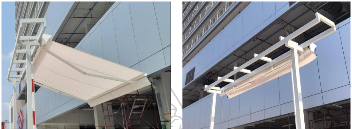
Figure 86 Movable awning shelter when it open
