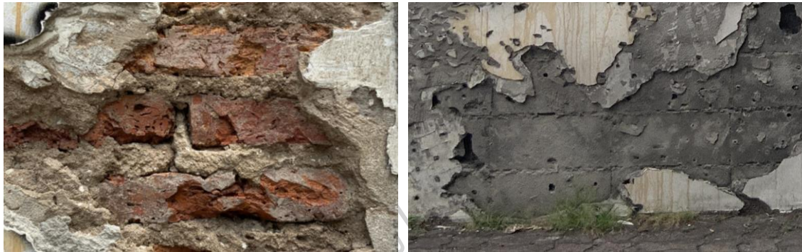
Figure 30 Brick masonry wall Source: Khakhanang Jonganurak (December 1, 2022)
