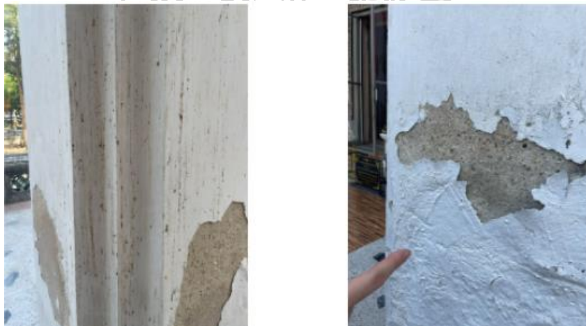
Dirt and bird drops on the column. The paint layer of the column peeled off.
