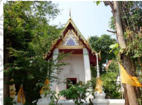
Fig. 65: Front photo of the south side small vihara , Wat Kampang , at Klong Bangjak canal on 3 rd March 2020.
