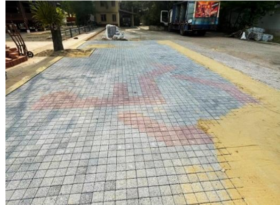
Fig. 83: A disabled parking lot using coloured pattern concrete block on packed soil, Wat Aranyigawas , Ratchaburi, on 6th April 2022.
