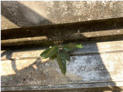
Fig. 66: The decoration wall of the ubosot with weed, Wat Kampang at Klong Bangjak canal during February 2023.
