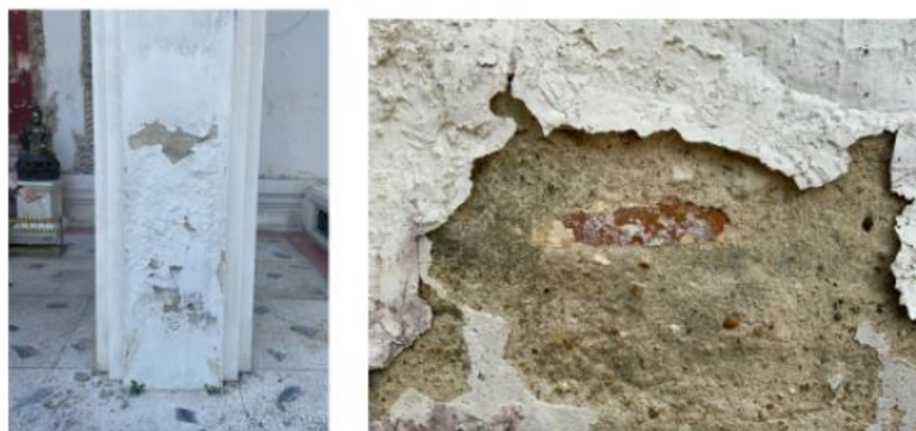
Dirt and bird drops on the column. The paint layer of the column peeled off.
