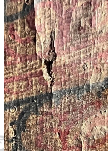
Fig. 77: Wooden door painting damage; abrasion, surface dirt, uplifting, and roof-shape, Wat Kampang at Klong Bangjak canal on 6 th February 2023.
