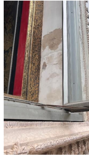
Fig. 67: The ubosot wall deterioration, Fig. 68: The ubosot wall deterioration around the window, Wat Kampang at Klong Bangjak canal on 6 th February 2023.
