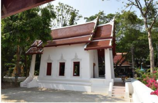
Fig. 62: Elevation photo of the north side small vihara , Wat Kampang , at Klong Bangjak canal on 3 rd March 2020.
