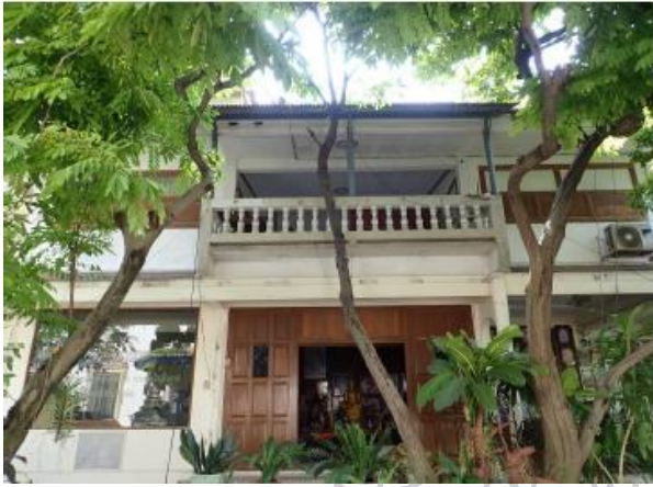
Fig. 45: Monk residence concrete building, Wat Kampong at Klong Bangjak canal on 3rd March 2020.
