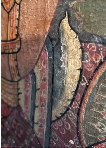
Fig. 75: Wooden door painting damage; dropping, flaked off, and surface dirt, Wat Kampang at Klong Bangjak canal on 6 th February 2023.
