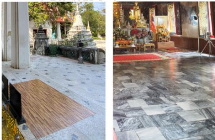
Terrazzo tiles at canopy of the ubosot . Marble floor inside the ubosot .
