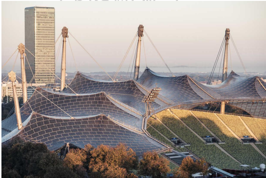
Figure 25 Munich Olympic Stadium Canopy in Munich, Germany, 1972.
