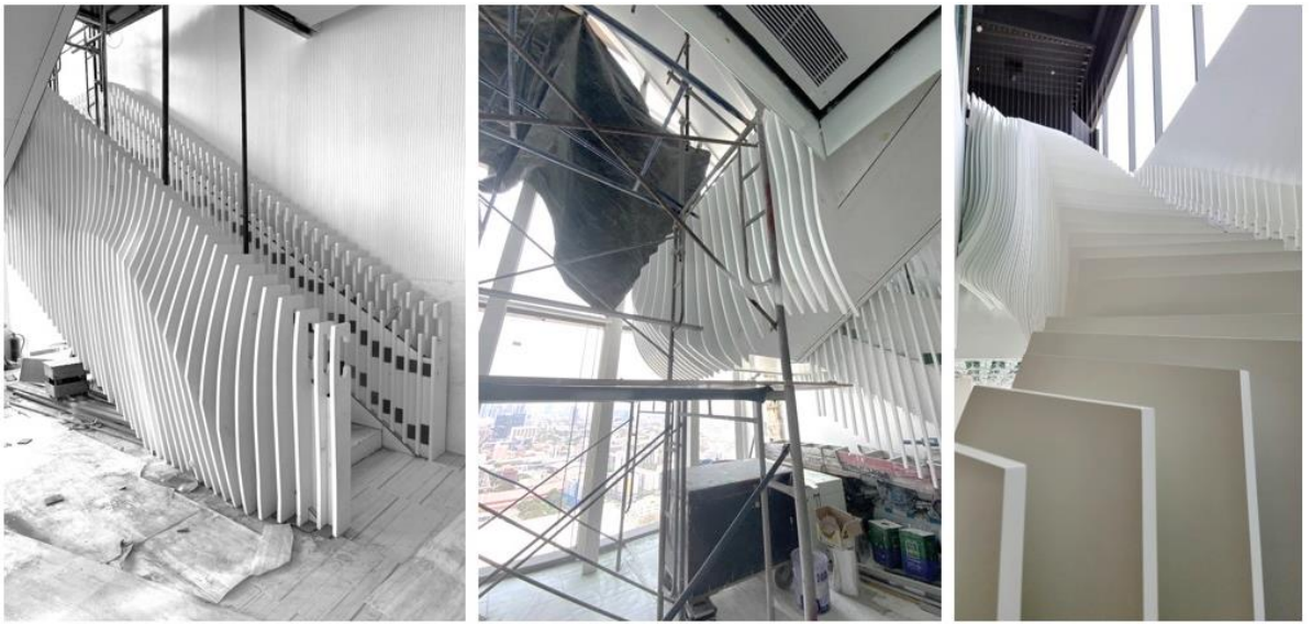
Figure 105 Process for Installing Parametric Stairs.
