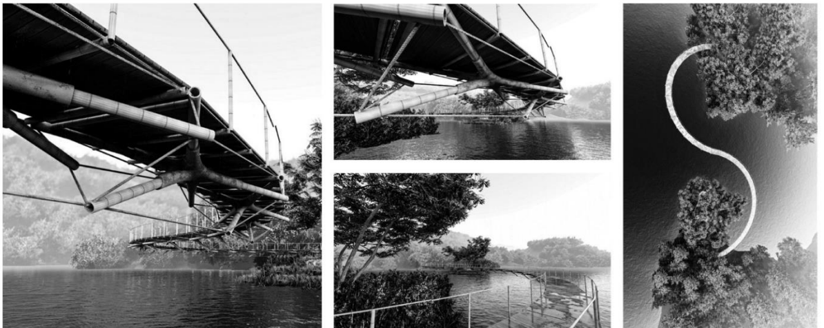
Figure 177 S Curve Bridge
