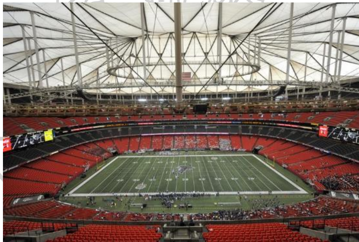
Figure 29 Georgia Dome by Levy and Weidlinger Associates
