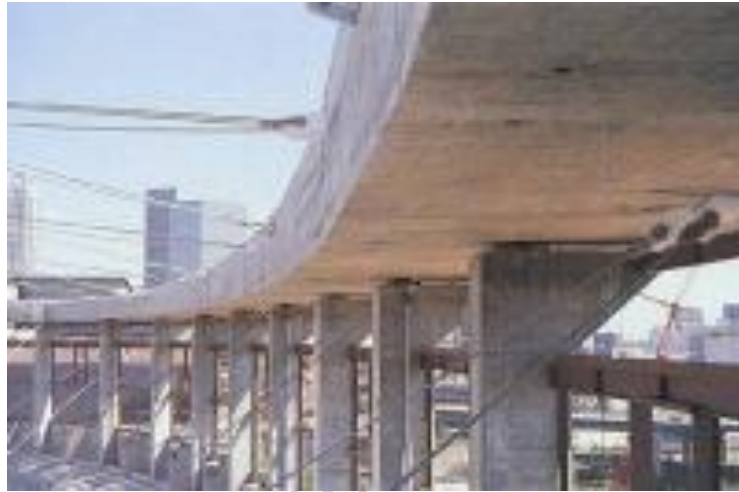
Figure 12 Georgia Dome by Levy and Weidlinger Associates
