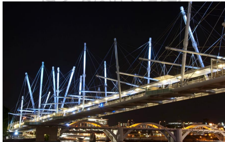
Figure 13 Largest tensegrity bridge in the world, Kurilpa Bridge, Brisbane.
