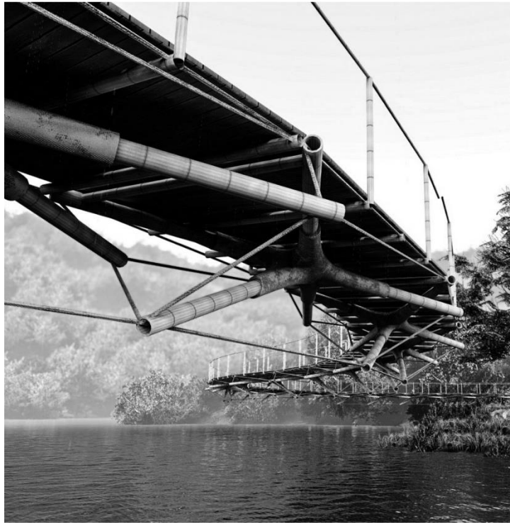
Figure 178 S Curve Bridge
