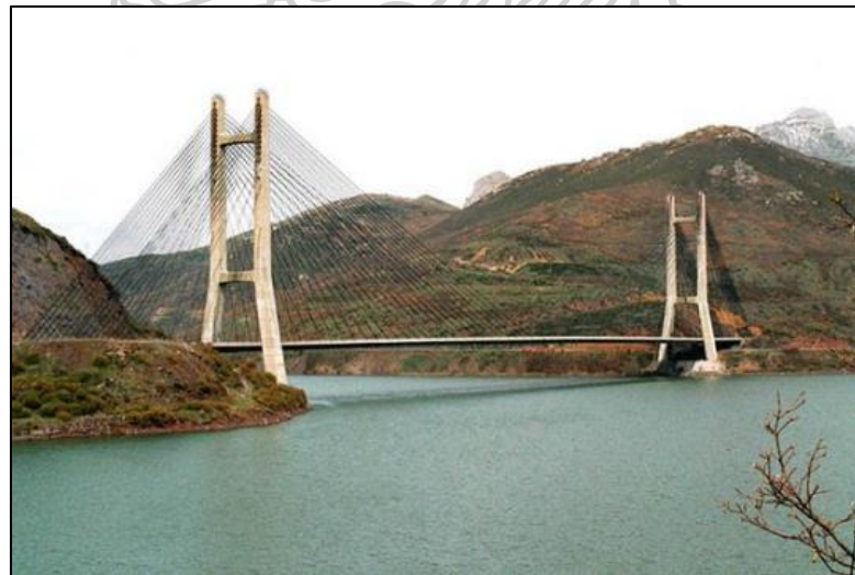
Figure 21 Barrios de Luna Bridge, Spain. Designed by Casado, built in 1983.
