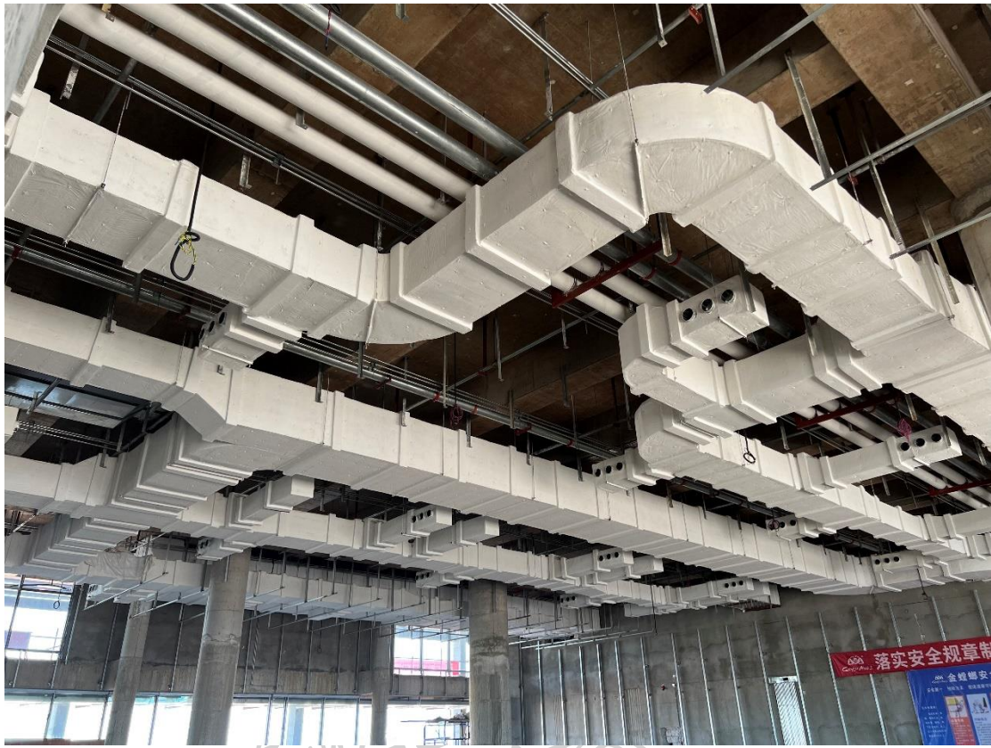
Figure 4.2 the insulation material
