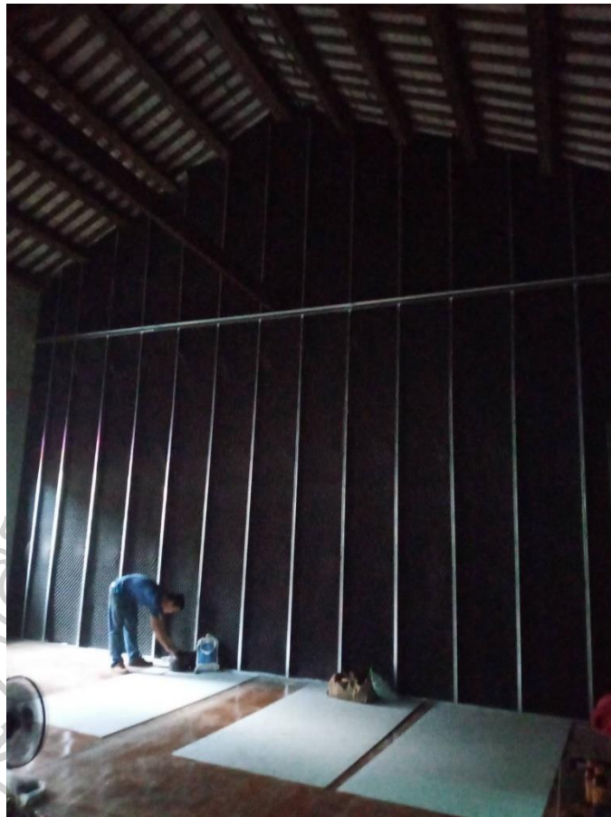
Figure 9 Inside of Artesia cafe/ noise cancellation wall installation
