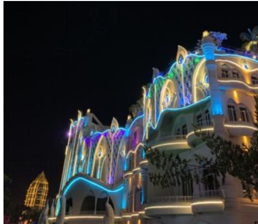
Figure 56: Exterior of Mekong River Jingland Hotel Source: The author in Mekong River Jingland Hotel (4 th November 2021)
