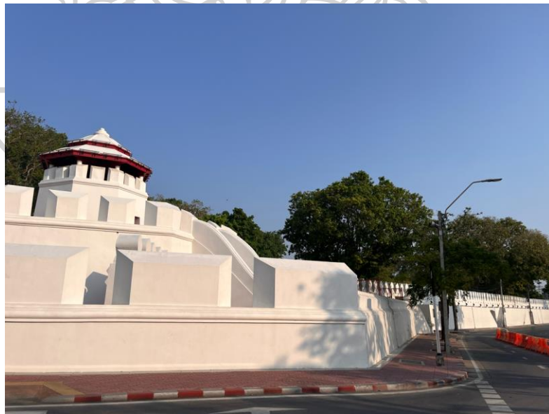
Figure 4: Continuous Wall of the Mahakarn Fort and its decorations Source: Mariia Lizunova, April 2024
