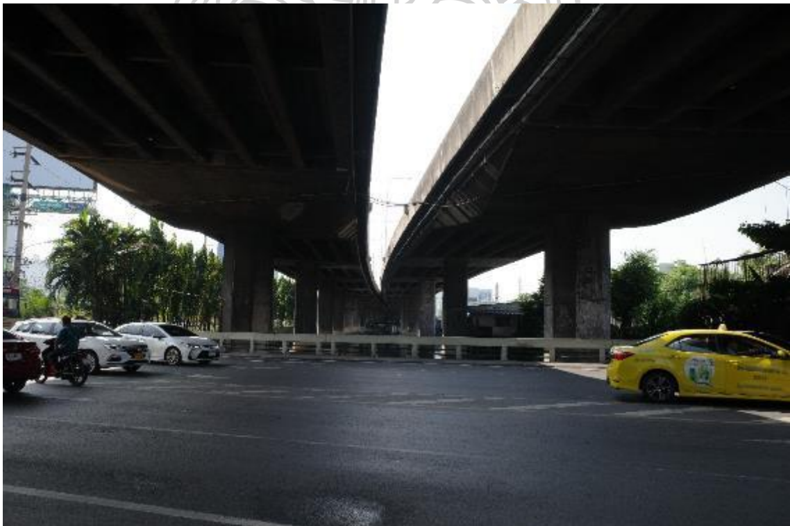
Figure 48 Highway lined along At Narong Rd.
