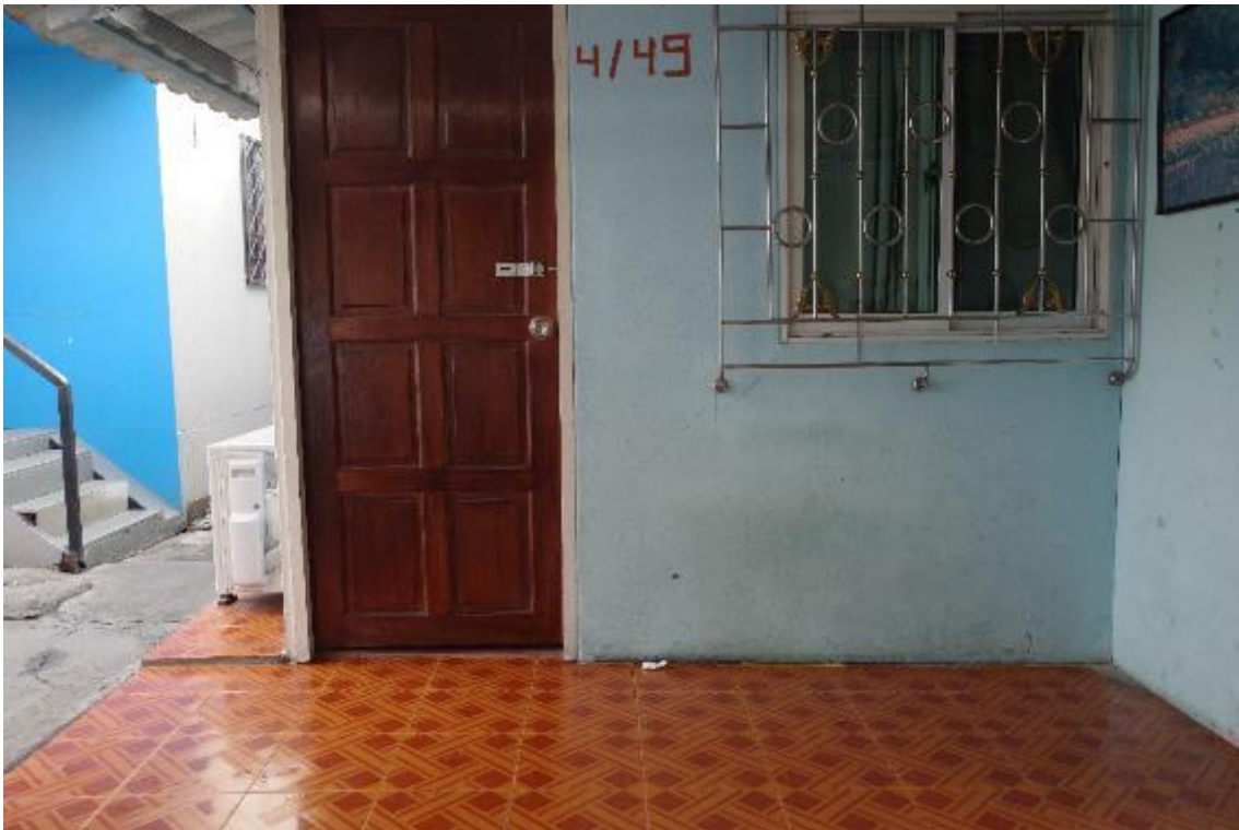
Figure 86 Frontage of HOUSE-02
