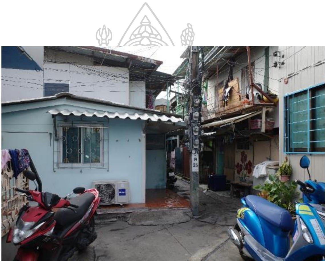
Figure 85 Roof added between HOUSE-01 and HOUSE-02
