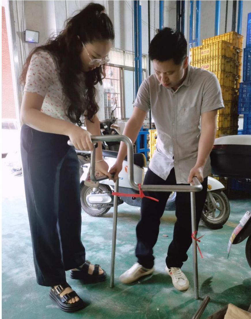
Figure 52 Main Framework of the Product after Welding
