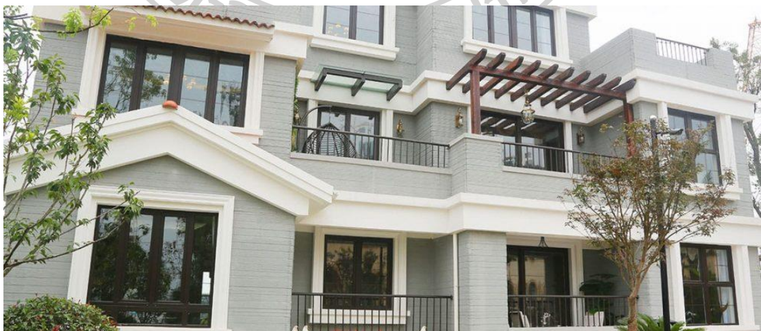
Figure 2.5 Residential buildings of WinSun.
