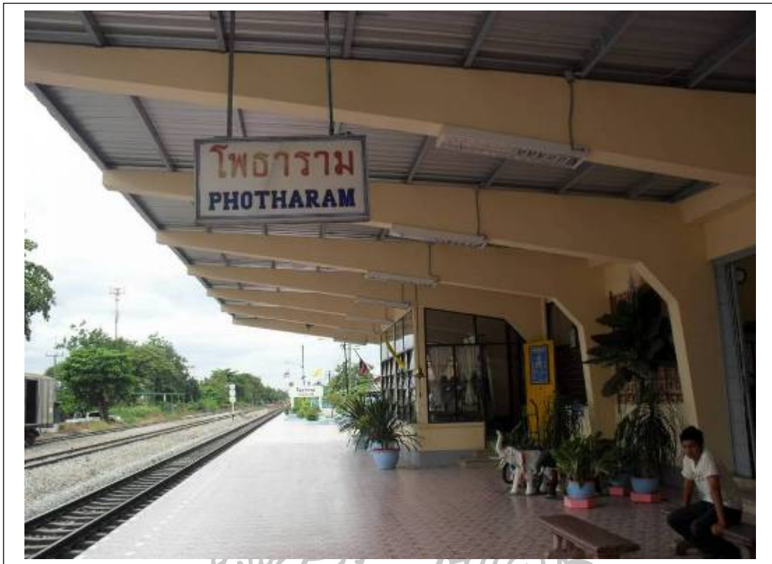
Figure 5 Photharam railway station
