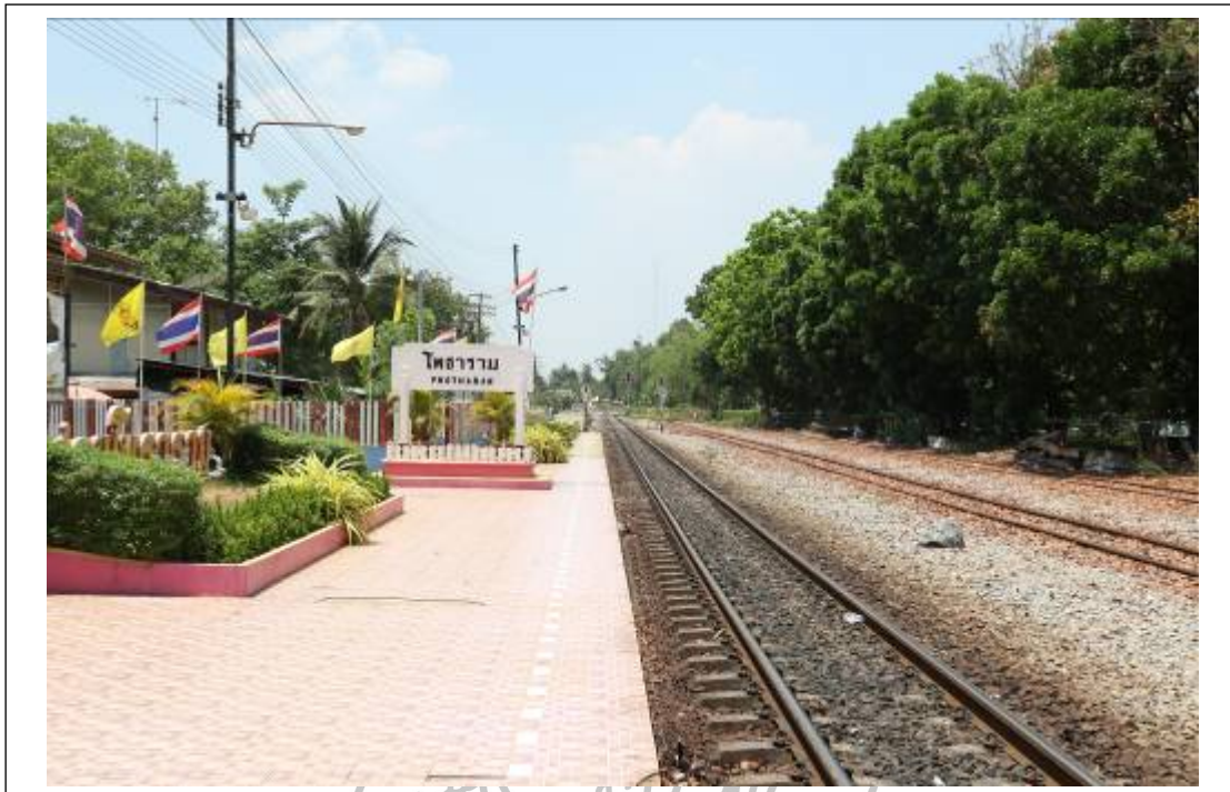
Figure 29 Photharam railway station
