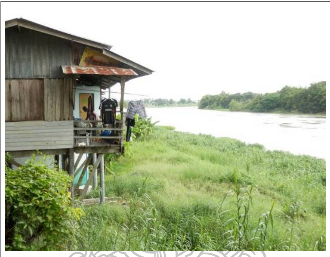
Figure 56 Elevated houses at Talad Bon
