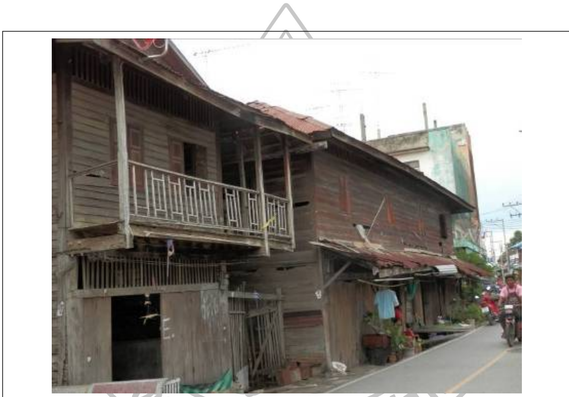
Figure 9 Character of buildings on Choekchai road at Talad Bon
