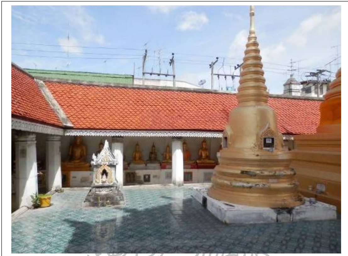
Figure 26 The cloister around the ubosot
