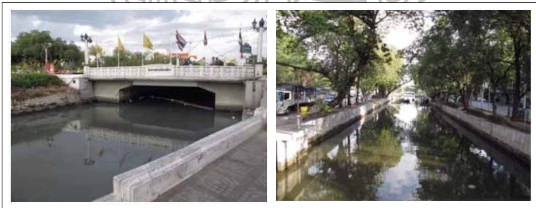
Figure 43 Khlong Khu Meaung Derm with concrete embankments and walkways along the khlong next to road
